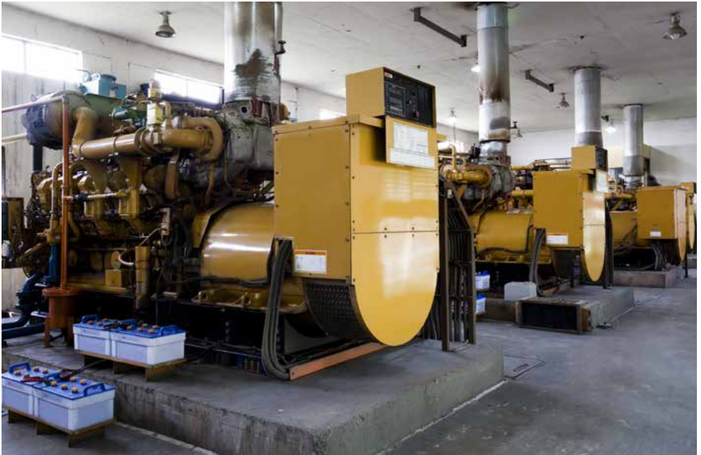
A standby diesel engine generator
